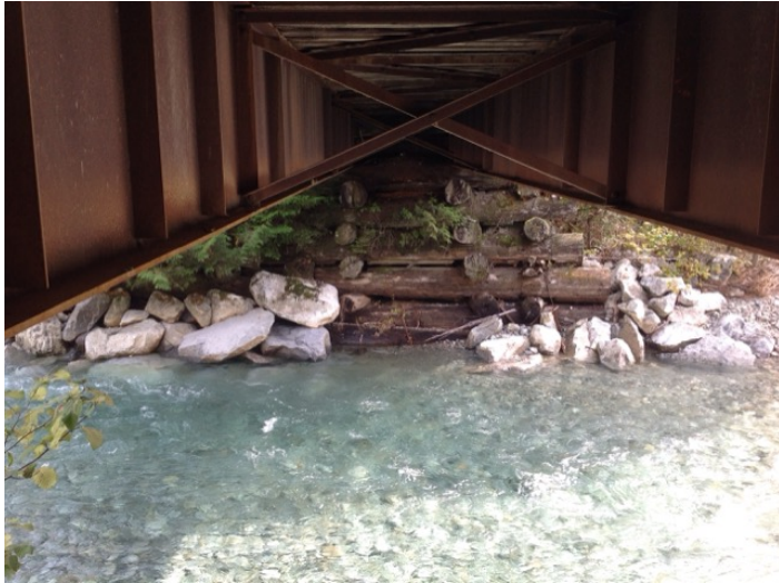
Left Bank Abutment when facing downstream
