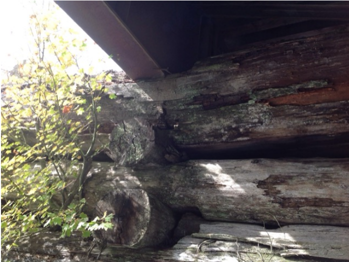
top crib log in pier
