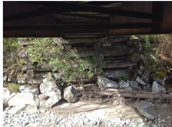
Right Bank Abutment when facing downstream
